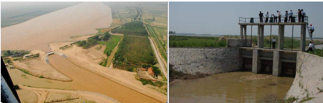
Diaokouhe River Ecological Water Diversion Program and Experiment of Restoring Water for the Old Course of Yellow River draws off water from Cuijia Water Control Project
